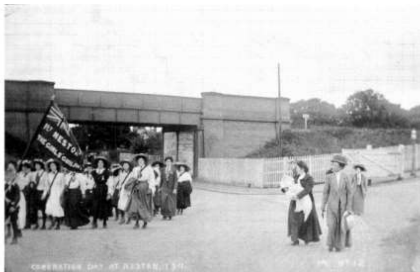
The former steel girder bridge across Station Road, Parkgate, built for the 1886 extension; the Girls Guildry procession was held as part of the local celebrations for the coronation of George V in 1911; the station entrance is to the right.
