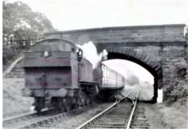
A West Kirby-bound train passes the same bridge in BR days pulled by a GW prairie tank loco. The right-hand track is the colliery branch.
