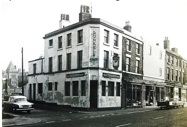
The Dunkeld Arms on the corner of Dunkeld Street (to the left) and West Derby Road in about 1974. This area has since been rebuilt.
