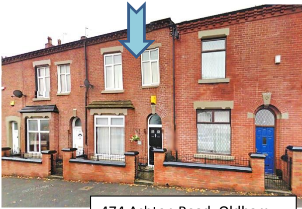
474 Ashton Road, Oldham [Source: Google StreetView]
