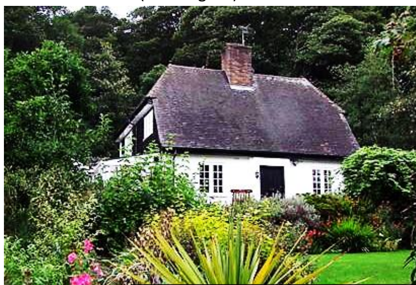
Rake Cottage, The Rake, Burton [Source : http://www.rightmove.co.uk/ ]
